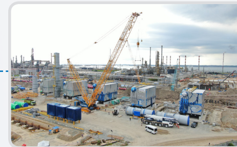
Delivery to Site 5 unit Steam Turbine Generator A-331-03 A-E
